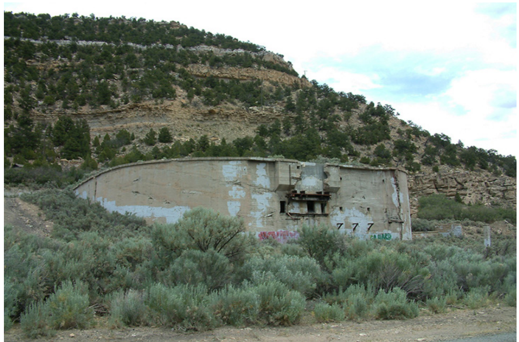
Standardville Coal Bunker
